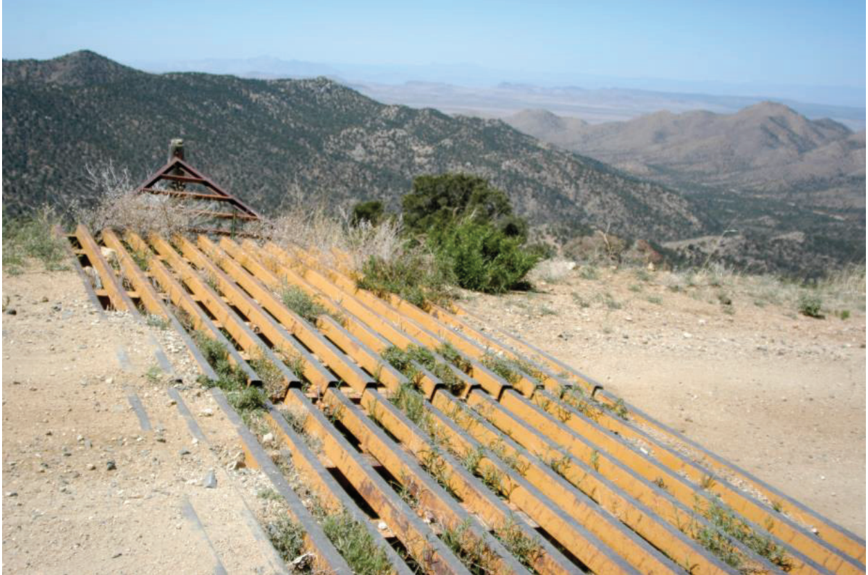
Cattle guard w/o rebars creates danger for mustangs. Cerbat ridge. Cerbat Mtn. HMA. 4/2018. Copyright by Craig C. Downer
